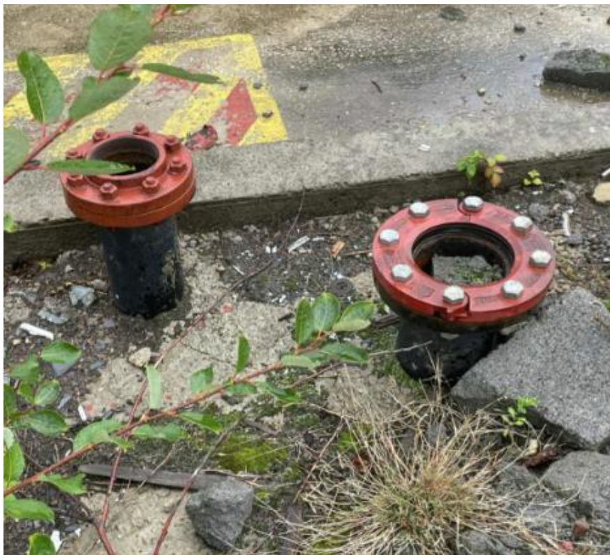
Relic pipework and concrete foundation
